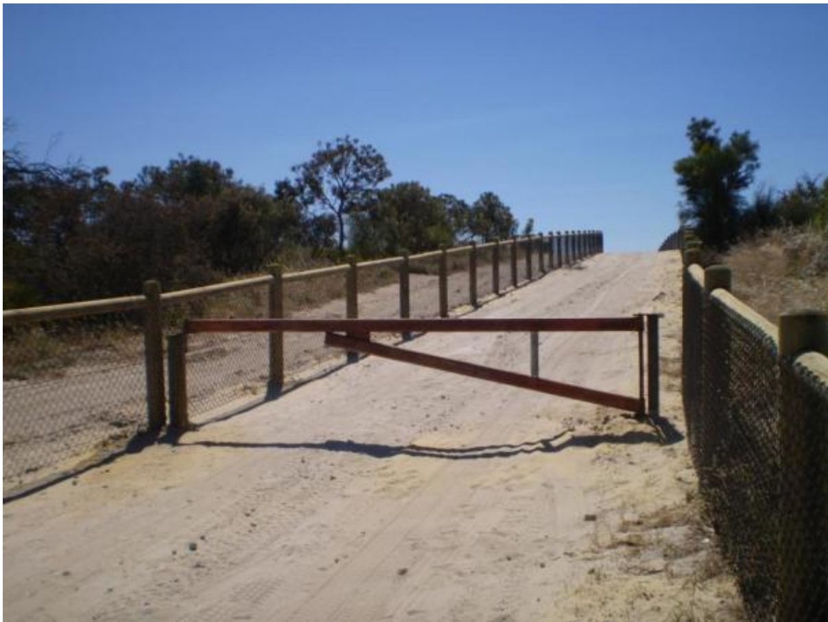
Plate 1: Example of access control fencing.
